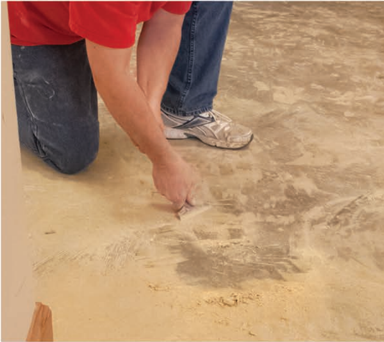
Removing mastic and glue when updating flooring can be a time-intensive process if manual scraping is required.
